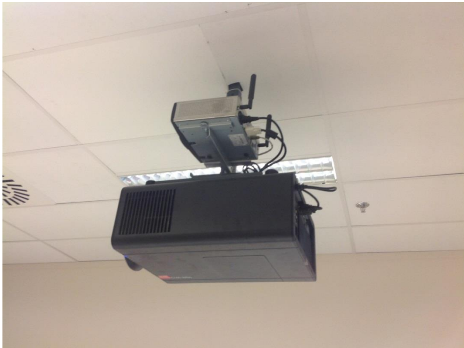
Figure 6: Example of correct ClickShare base unit installation
