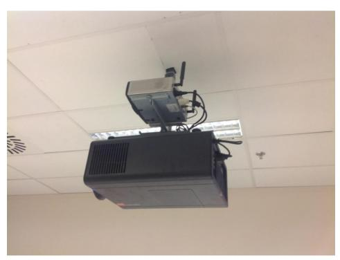
Figure 6: Example of correct ClickShare base unit installation
