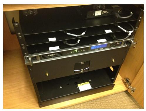
Figure 8: Example of wrong ClickShare installation: the antenna are not connected on the ClickShare rack-mounted kit
