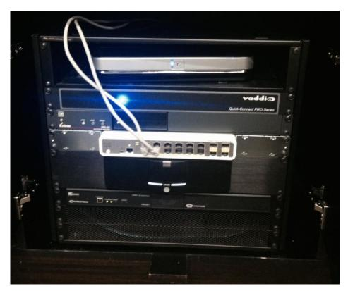
Figure 9: Example of wrong ClickShare installation: an incorrect rack-mounted kit is used and the ClickShare base unit antennas are enclosed in the shelf
