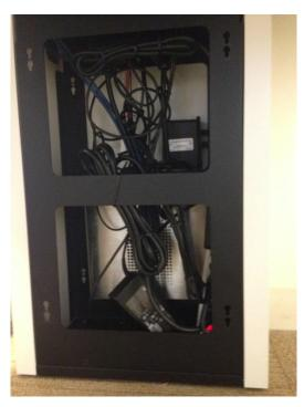
Figure 10: Example of wrong ClickShare installation: the base unit is placed inside a metallic closet without using antenna extension kit which strongly deteriorates the signal quality
